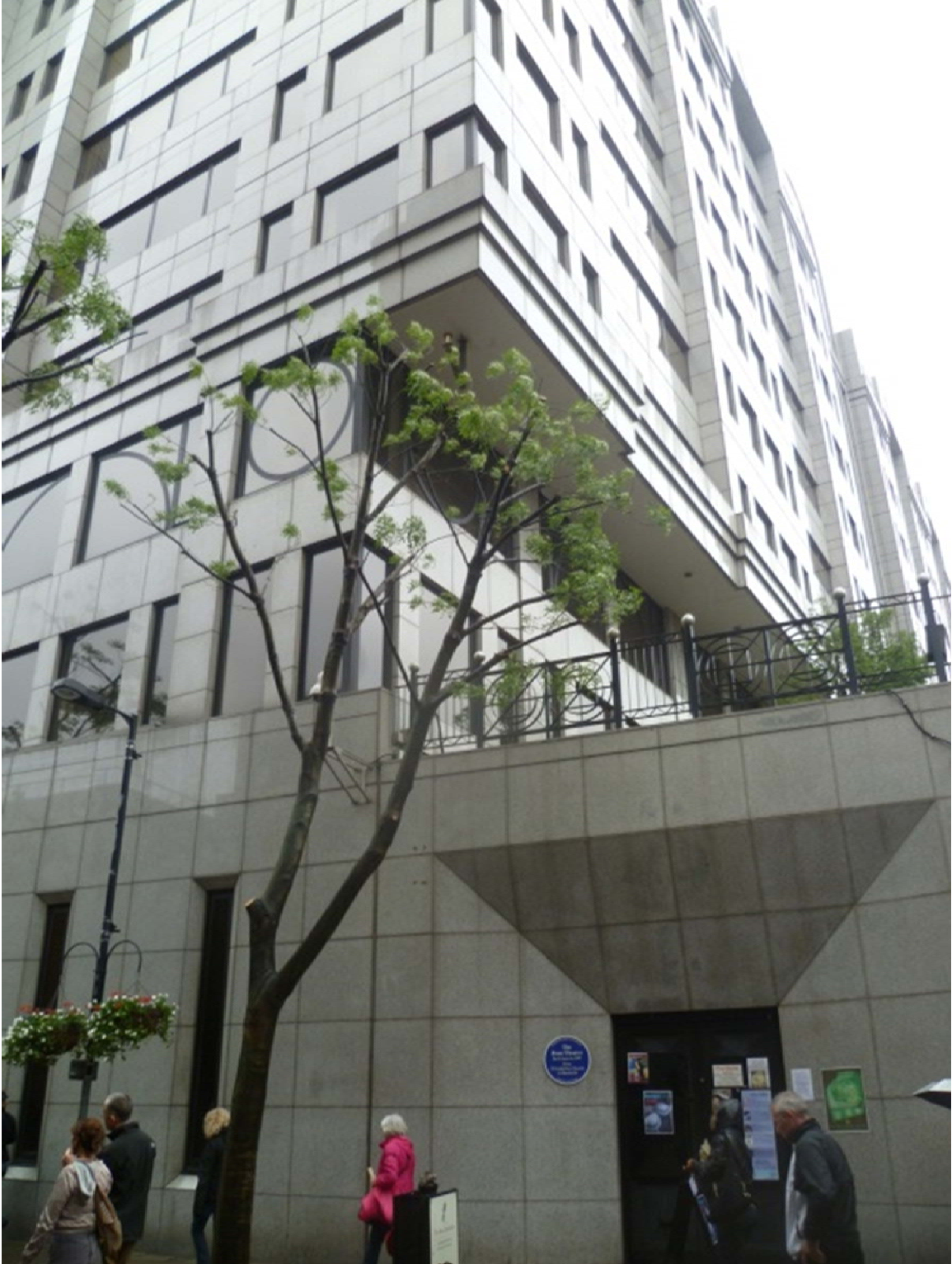
Figure 2.9 Picture of the Rose Theatre building as it stands now (Picture taken in June 2012). The door on the bottom right hand leads to the basement where the theatre remains are preserved.
